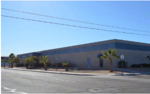
1310 S. 3rd Ave., Yuma. Photo Credit: City Feet
